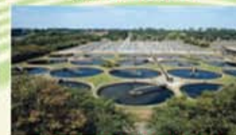
Sewerage Treatment Plant
