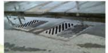
Storm Water Drainage - 4.5 Kms.
